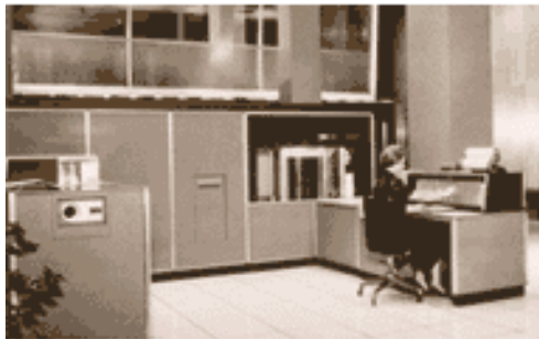
The first hard-disk drive, IBM's RAMAC 350 (top), stored 5 million characters on 50 24-inch disks. Announced in May 1955, the drive, with vacuum-tube control electronics, was part of the RAMAC 305 system (bottom).
